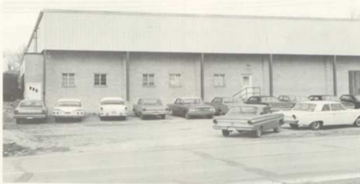
Winkler Warehouse is shown above after new addition is completed
