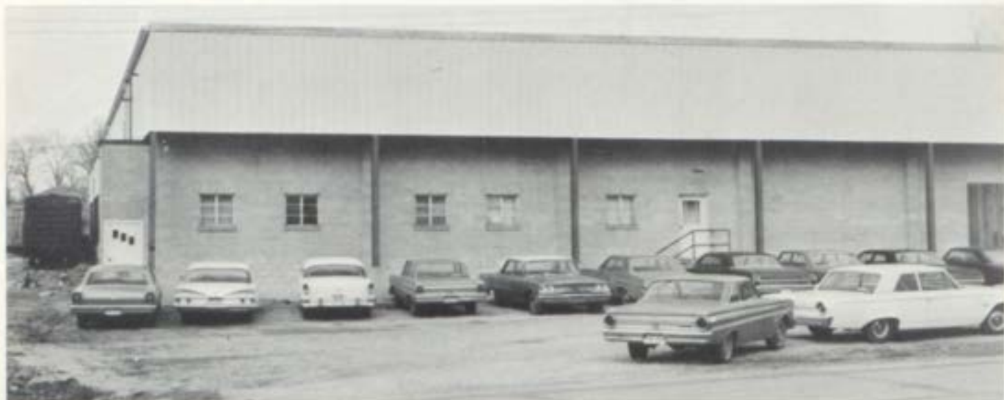
Winkler Warehouse is shown above after construction of the new addition is completed.
